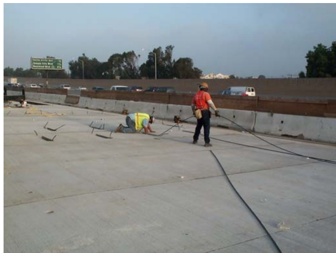
Continuous installation near El Monte, Calif. (2004)
