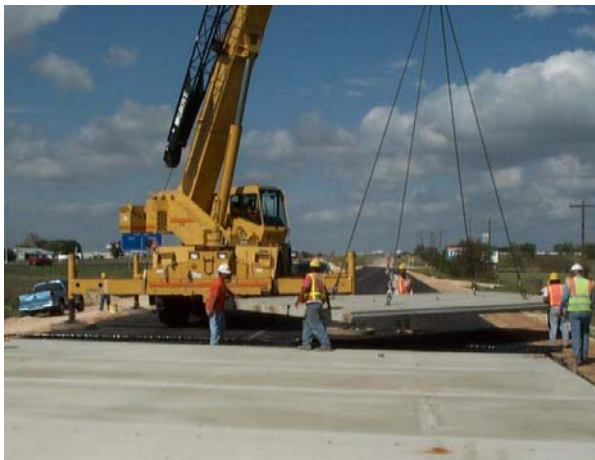
Continuous installation near Georgetown, Texas (2002)
