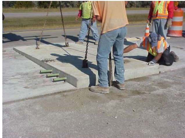
Intermittent installation on I-675 near Detroit (2003)
