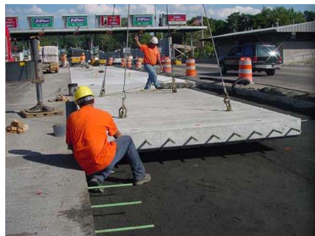
Continuous installation at the Tappan Zee Bridge Toll Plaza, Tarrytown, N.Y. (2001)
